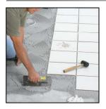
Use to adhere tile and backer board to subsurface
