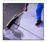
Seal seams, fill cracks and holes, and level floor before installing tile
