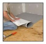
Use in wet areas to prevent moisture from damaging subsurface
