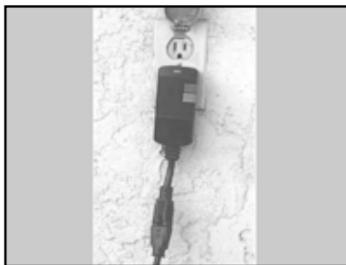
(E) Unplug the GFCI from the power source
