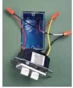
from the fan to the switch; however, the previous installer may not have marked it. If unmarked, wrap tape around its end and splice it with the switch's black lead. Splice the red wire (from the light) and the black wire (from the fan) to the switch's light and fan leads.
