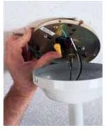
against the canopy when the fan is running. Clip the canopy onto the mounting plate and tighten the screws.
