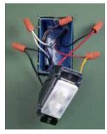
manufacturer's instructions; wire colors vary. Most likely you'll splice the black wire bringing power to the black switch lead, and splice the two white wires together. Then splice the black wire from the fan and the red wire from the light to the switch's fan and light leads.
