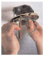
bolts are provided, push each one through the mounting plate as shown. When both bolts are in place, tighten the plate onto the ceiling.
