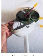
motor) and the blue or striped lead (for the light) to the black house wire, and the white lead to the white house wire. If you have three-wire cable, connect black to black, white to white, and red to the blue or striped light lead. Check the manufacturer's directions. You may choose to install a remote control unit.
