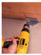
Buy a new-work ceiling fan box with a brace. Slide the box along the brace to position it. Tighten the clamp. Attach the brace by driving in 1-1/4-inch wood screws.
