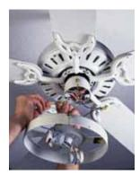
the light kit leads. Screw the light kit up to the fan. Some light kits require a spacer ring between the fan and the light. The spacer ring should come with the kit or the fan.
