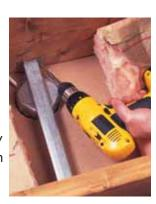
**USE A FAN-RATED BOX.** A ceiling fan box is different than an ordinary ceiling box in two ways: First, it's designed to attach firmly, either directly to a joist or with a support bar. Second, it's equipped with deep-threaded holes or strong bolts so that you can tightly clamp the fan to it. You'll never get this kind of strength from an ordinary ceiling box.
