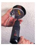
box, and clamp the cable to it. Hold it in place and drill pilot holes; then drive in 2-inch wood screws. (Don't use drywall screws or all-purpose screws—they break too easily.)
