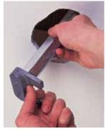
through the hole and spread until it touches the joists on both sides. Make sure the the legs of the brace rest on top of the drywall or plaster.
