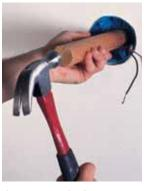
get to fasteners. If the box is nailed to a joist, cut around the box to enlarge the hole, and tap the box loose using a piece of wood and a hammer. You may be able to cut through fasteners with a reciprocating saw or a metal-cutting keyhole saw. Take great care not to slice through any cable.
