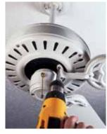
faces down. Attach each bracket to the motor with two screws. Drive the screws slowly to avoid stripping. Don't bend the brackets as you work.
