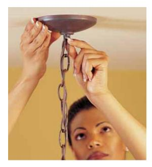
HANG THE FIXTURE. Thread the fixture's mounting stem into the mounting strap on the ceiling box. Although the fixture is now securely hanging from the ceiling, the box and mounting hardware are still visible. Slide the canopy up against the ceiling to cover the mounting hardware; tighten the locknut against the canopy.
